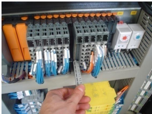
Figure 30: Connection of the system management encoder 系统管理编码器的连接
