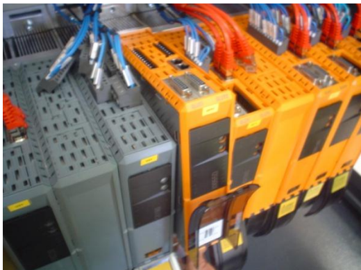
Figure 87:Replacing a drive 更换驱动器
