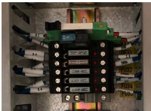
Figure79:Replacing fuses 更换熔断器
