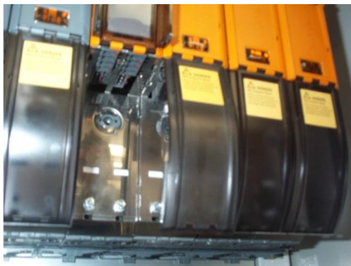
Figure 84: Replacing a drive 更换驱动器
