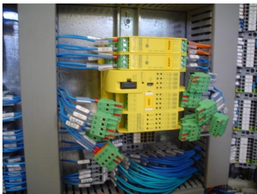
Figure96:Replacing the safety PLC 更换安全 PLC
