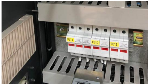
Figure78:Replacing fuses 更换熔断器
