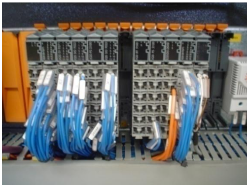
Figure 30: Connection of the system management encoder 系统管理编码器的连接
